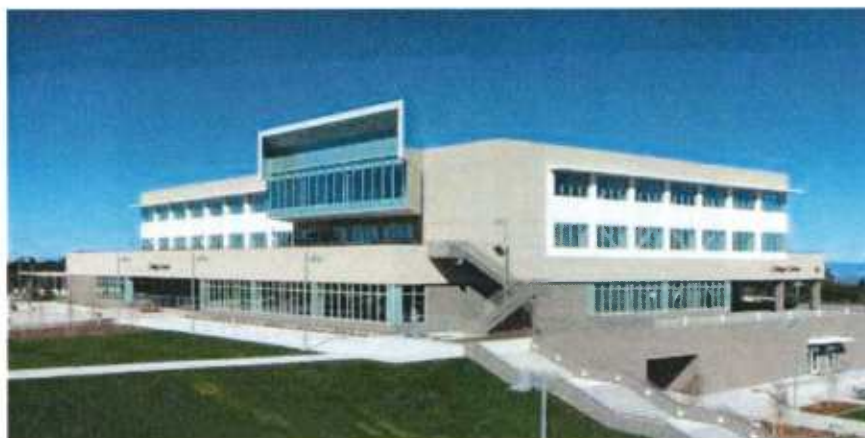
(AR1:490 [new Building 10 College Center])
